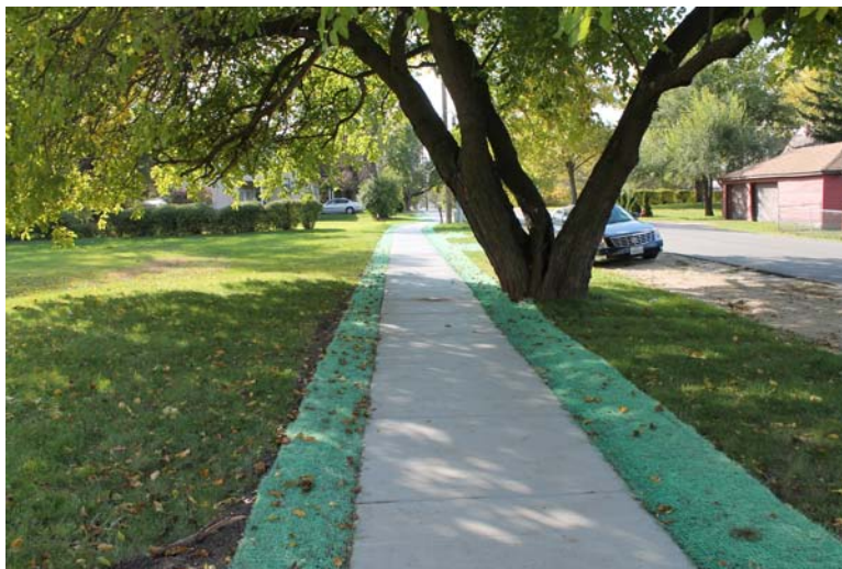
A "Safe Routes to School" grant provided the funding for Fairmont's first sidewalks located in front of Fairmont School.
